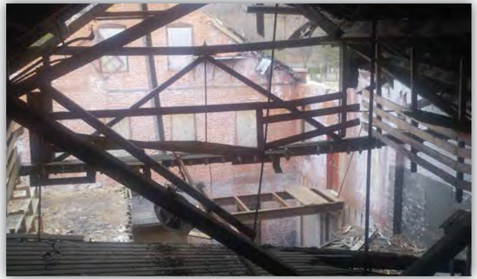
The Match Factory space as it was in 2010 during demolition.
