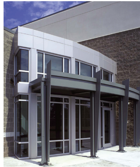
Non-structural steel columns outside the employee entry are more than purely decorative, they will prevent a vehicle intrusion. The double-height window gives the illusion of a single-story building, creating a more human scale near the entrance.
