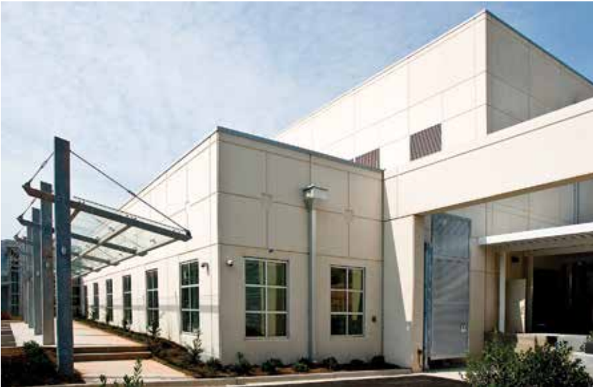
The precast concrete panels cladding the building were typically 12 feet wide and 37 feet tall, with blockouts for ventilations ducts and other HVAC needs added on the second level. Photo: Metromont Corp.
