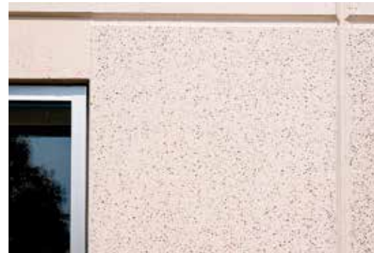
The panels feature an off-white face mix with a light sandblasted finish, which matched the finish on the original building erected four years earlier by the same design and construction team. Photo: Metromont Corp.
