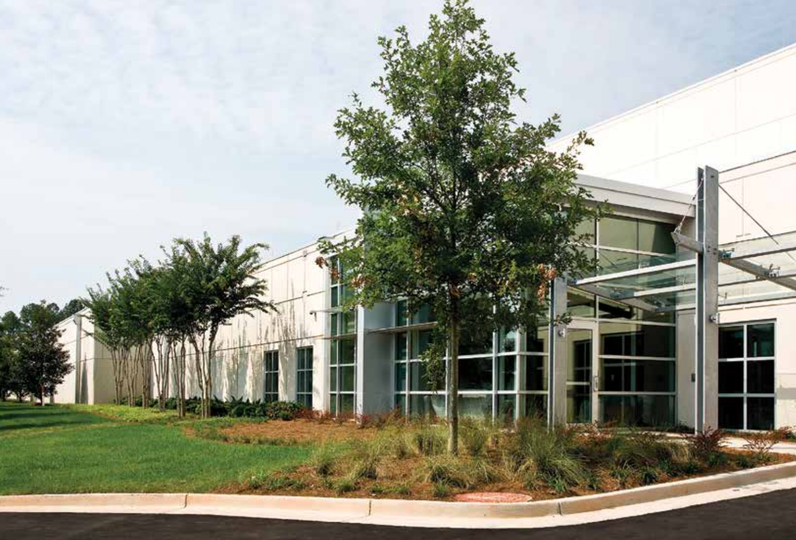
The building's first floor features offices, while the processing equipment was placed on the second floor, with no windows interrupting the panels. Photo: Metromont Corp.
