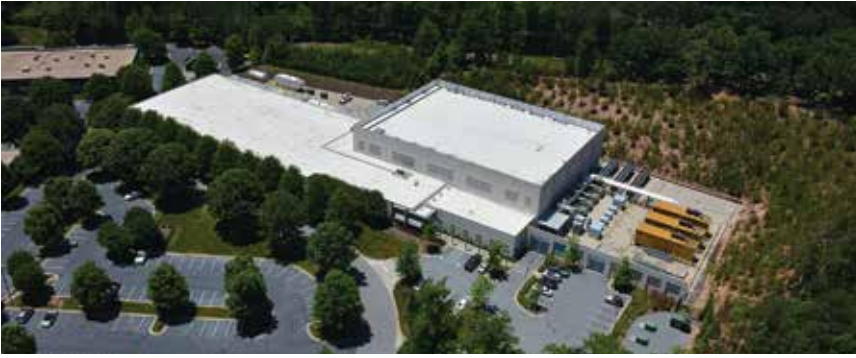
The new 60,000-square-foot addition (square building) was set against the existing 70,000-square-foot longer building to allow the original lobby to serve both facilities, maximizing space for data processing. Photo: Aerial Innovations of Georgia.
