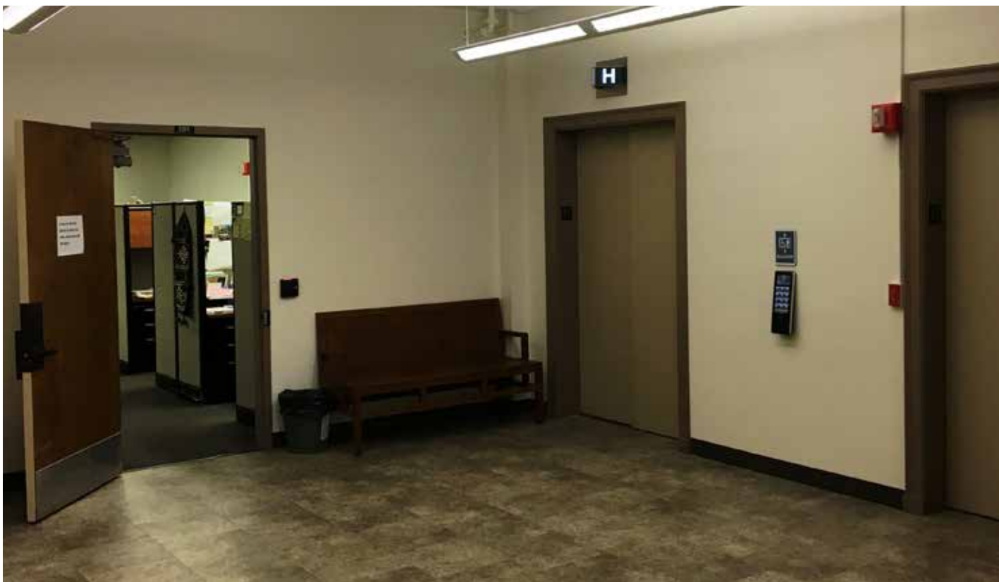
Existing elevator lobbies served only as secured access points. Photo by Pieper O'Brien & Herr Architects.
